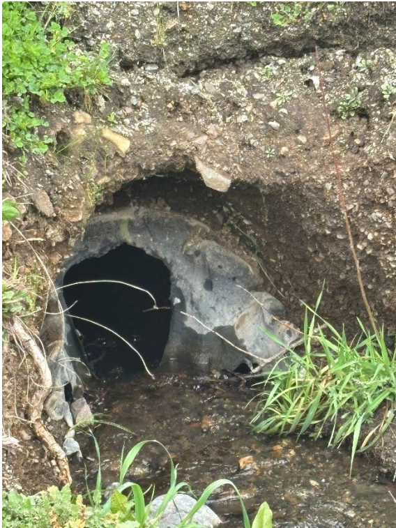
Photo 8. The culvert under the bike path at Blue Heron Park.
