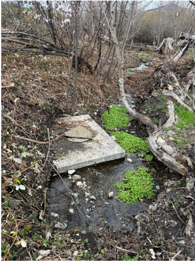
Photo 13. Looking downstream at the bike path culvert on the Unnamed Tributary to Bear Creek.
