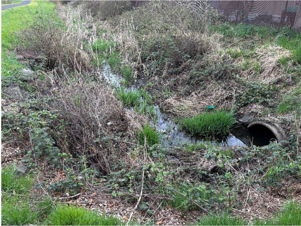
Photo 3. OR99S culvert outlet on South Stage Road
